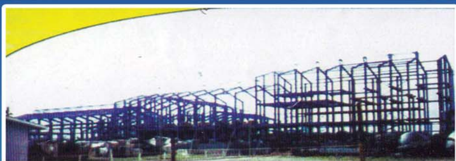
STEEL STRUCTURE SUGAR MILL, OKKAN (MINISTRY ONE)
