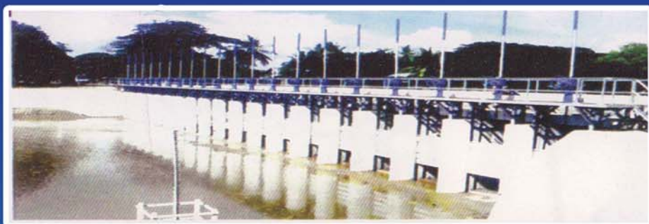
AHBYA SLUICE GATES PEGU DIVISION (IRRIGATION DEPT)
