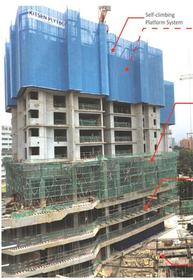
Aluminium System Formwork
