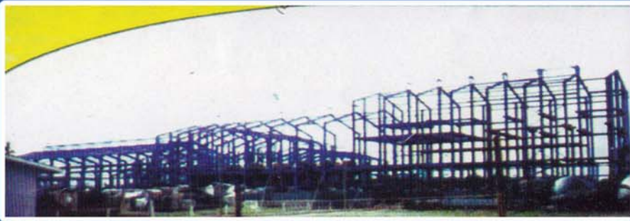
STEEL STRUCTURE SUGAR MILL, OKKAN (MINISTRY ONE)
