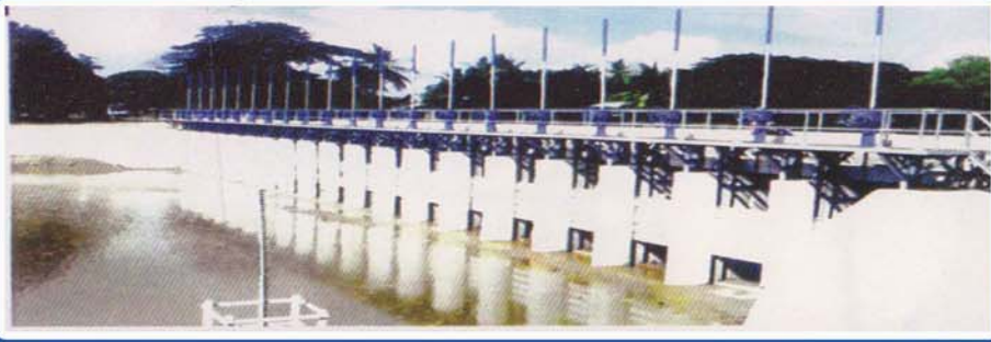
AHBYA SLUICE GATES PEGU DIVISION (IRRIGATION DEPT)
